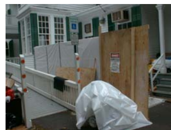
Asbestos abatement enclosure.
